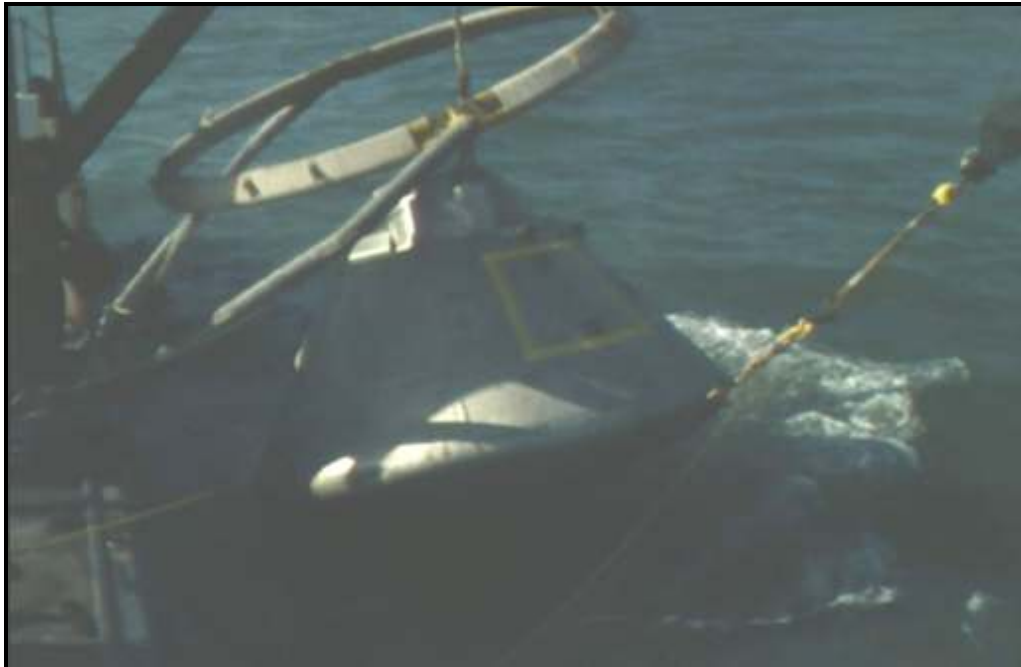
Photo #10: Block II BP-1101A being deployed during unmanned Apollo Block II uprighting system test in 1967 from MV Retriever in Gulf of Mexico (Photo Credit: Still from NASA FR-S67-008 DVD).
