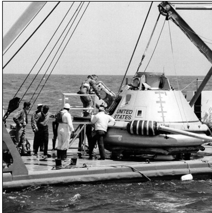
5. CM-007A onboard M/V Retriever in Gulf of Mexico prior to Block II 48-hour manned postlanding systems qualification test with astronaut crew (James A. Lovell, Jr., Stuart A. Roosa, and Charles M. Duke, Jr.) on April 5-7, 1968 (Photo Credit: NASA S-68-31882)
