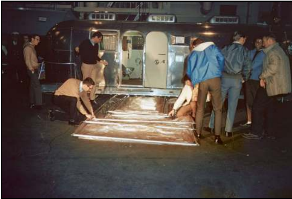
8. JSC recovery engineers prepare transfer tunnel prior to erecting in USS Guadalcanal hangar deck on March 3, 1969. (Photo Credit: NASA)
